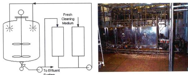
Figure 4: Cleaning in Place
